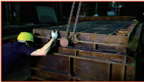
4 | 型被せ Mold Assembling
